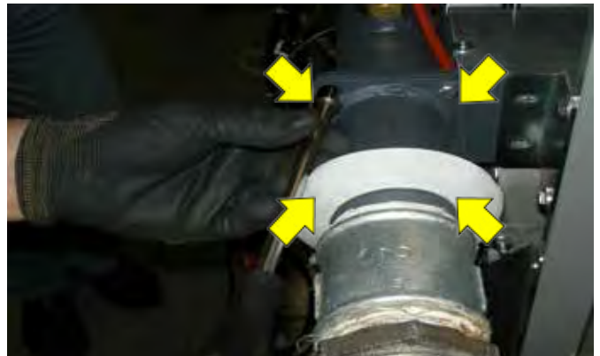
- Remove the four screws with a 10 mm socket wrench, then the gas flange
